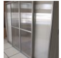
Cold Aisle Containment System with door at the front and the end of the row
